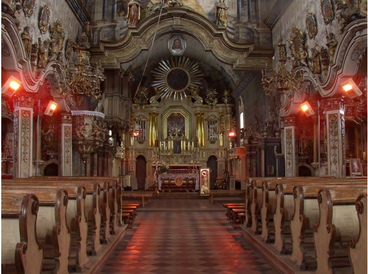
Fig. 2. Wooden church of St. Michael Archangel in Szalowa, Poland. View of the interior with overhead radiant electric heaters operating.
