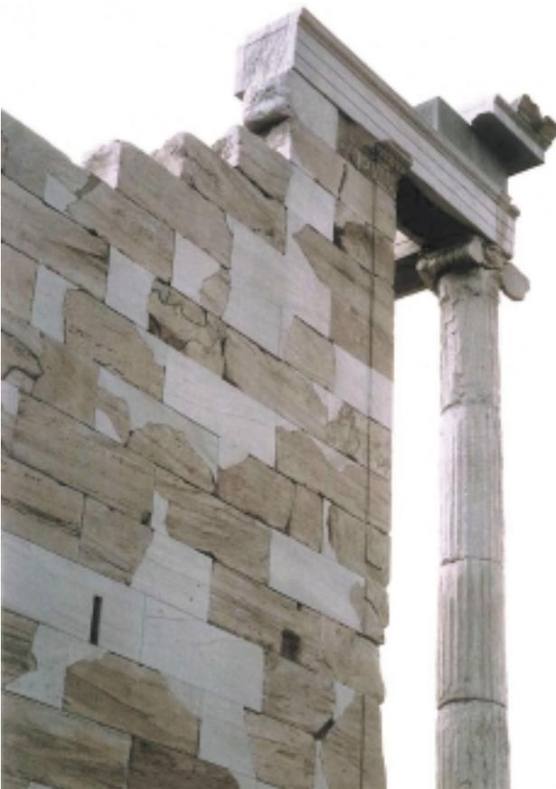
**Figure 2.** A fragment of the restored Acropolis (Athens), with original marble blocks as well as the Pentelic marble recently inserted to restore the architectural structure. The ancient marble pieces are bio-patinated, while the replacements still possess the colour of freshly quarried marble.
