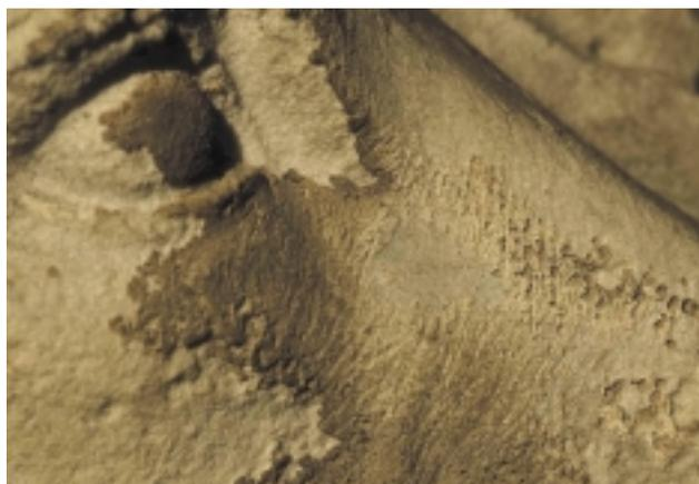
**Figure 7.** The skull of a horse at the Colonna Traiana in Rome. The horse skull (and especially the eye) exhibit (1) surface loss resulting from pollution and acid rain, and (2) different stages of bio-patina formation and bio-pitting of the patina as well as the original rock.
